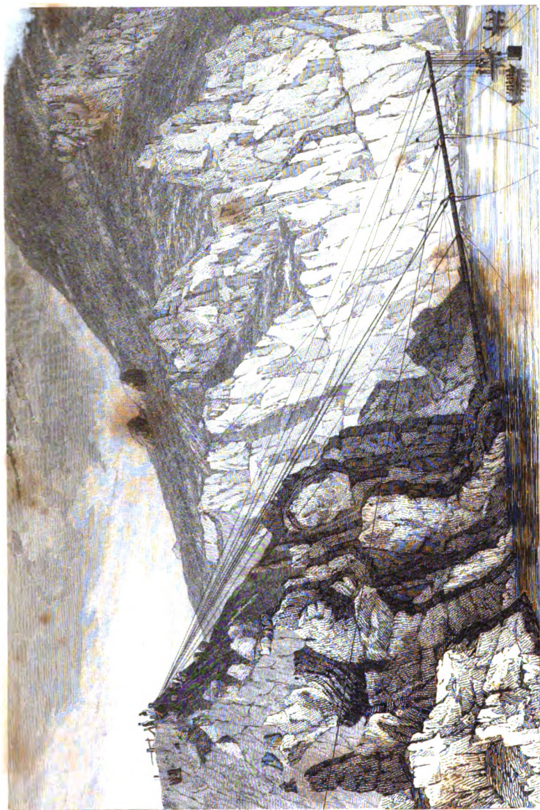
Cap. T. Dickinson's method of recovering the Treasure from the Wreck of the Thetis, at Cape Frio.
